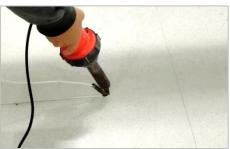
Welded seams must cool to room temperature before trimming in two steps, rough and fine trimming.
